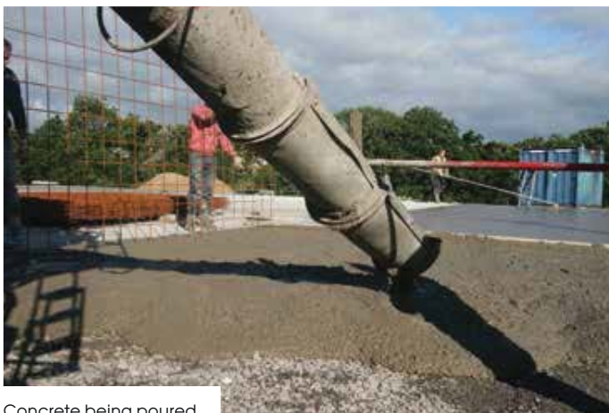
Concrete being poured
