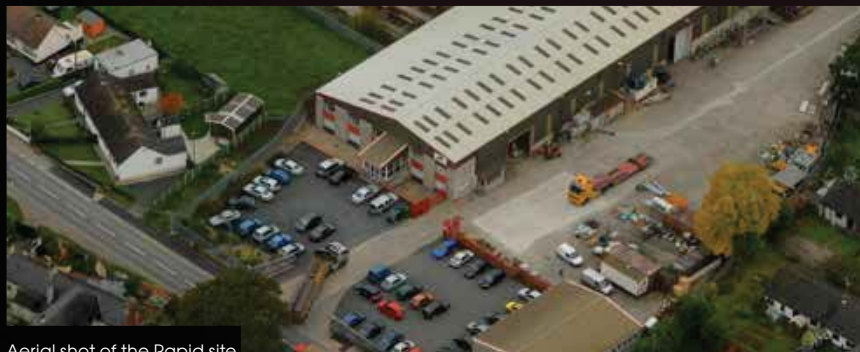
Aerial shot of the Rapid site
